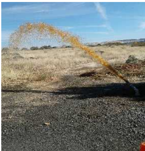
< Blow Off being flushed on Sunridge Ave.
